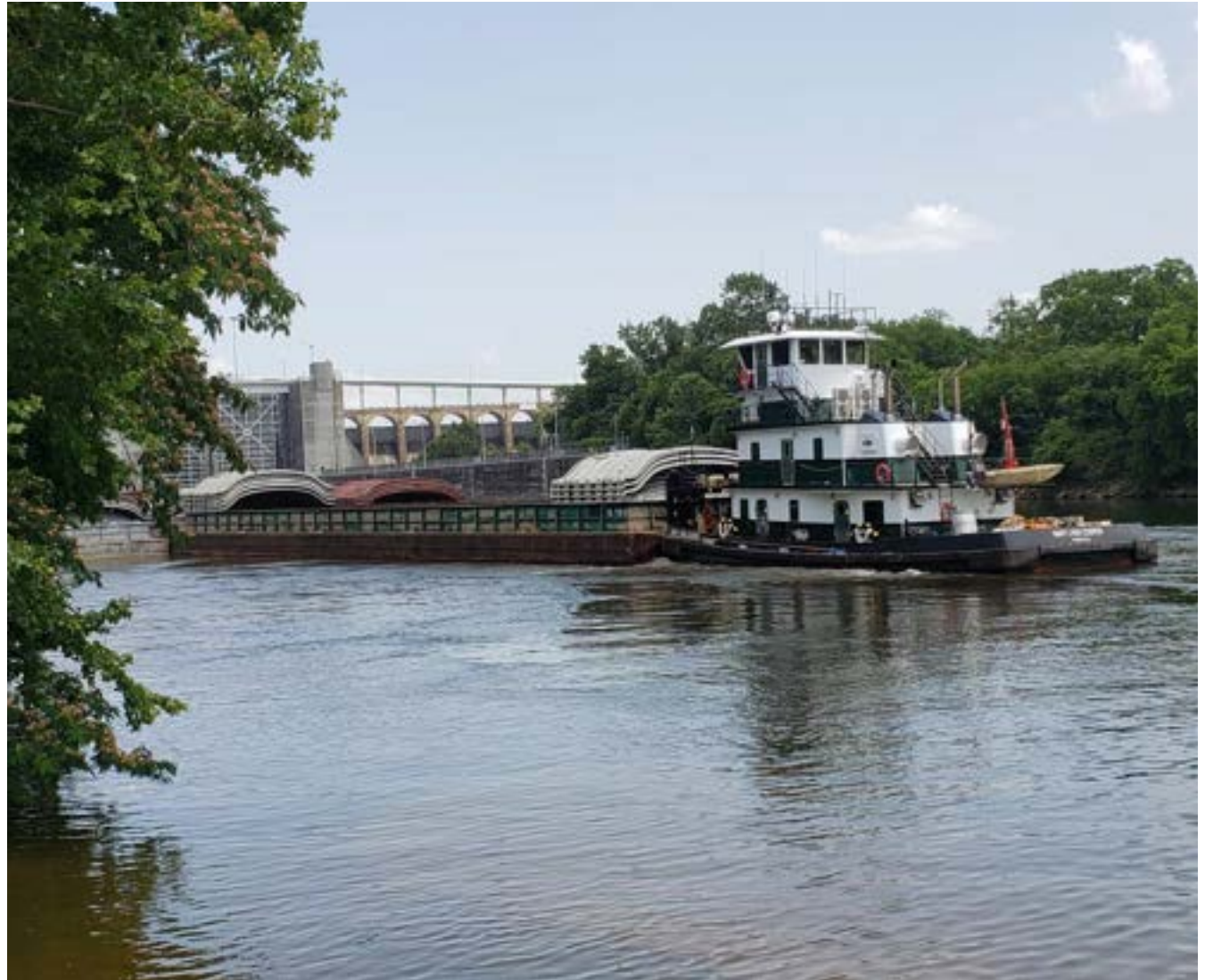
Wilson Lock and Dam - Florence, Alabama
