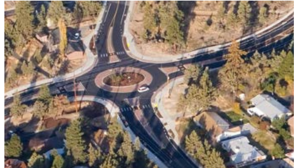
This roundabout features designated ramps that transition people on bicycles from the bike lane on to a shared use path or wide sidewalk. People on bikes are then directed back on to the roadway, or across a marked crosswalk. Crossings are set back from the circulatory lane and orient people walking and on bikes so that they are better able to see oncoming cars.
